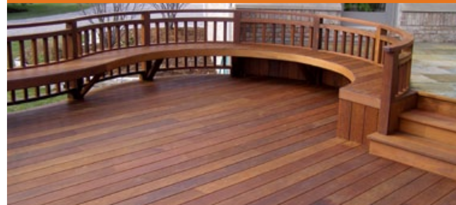
Standard Decking (Ipe Shown - Plug Method & Face Screw)
